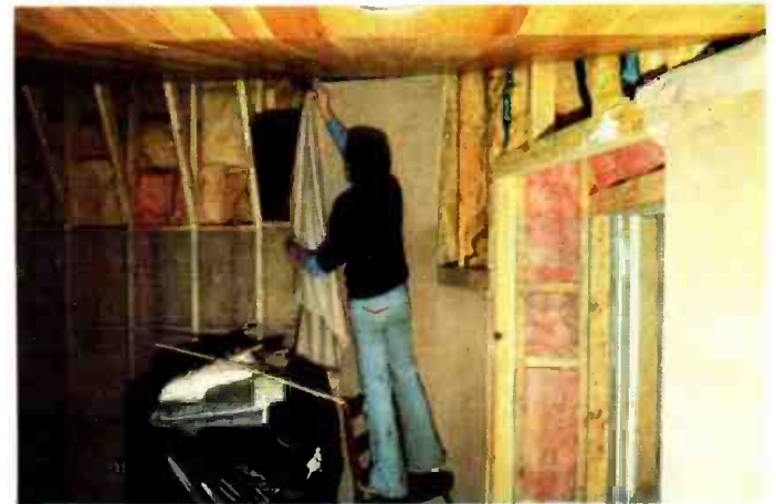
Hanging the corduroy over the rear control room wall.
