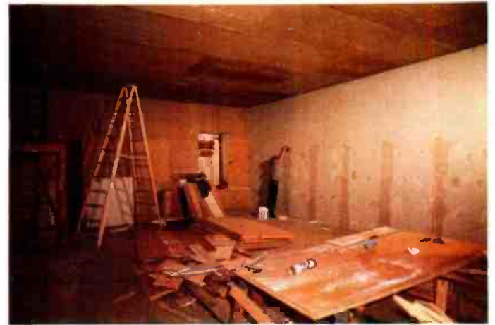
Taping and caulking gypsum layer over sound deadening board in studio.
